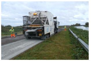
2 crews worked over the weekend to meet the deadline. The area of the road showing severe movement which covered an area of 500m2 was planned out to an addition 250mm in depth. This material was stockpiled on site.
