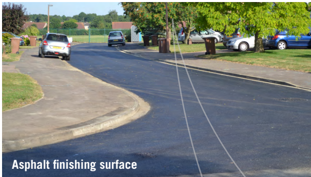
Finished recycled layer after application of emulsion and bituminous grit
