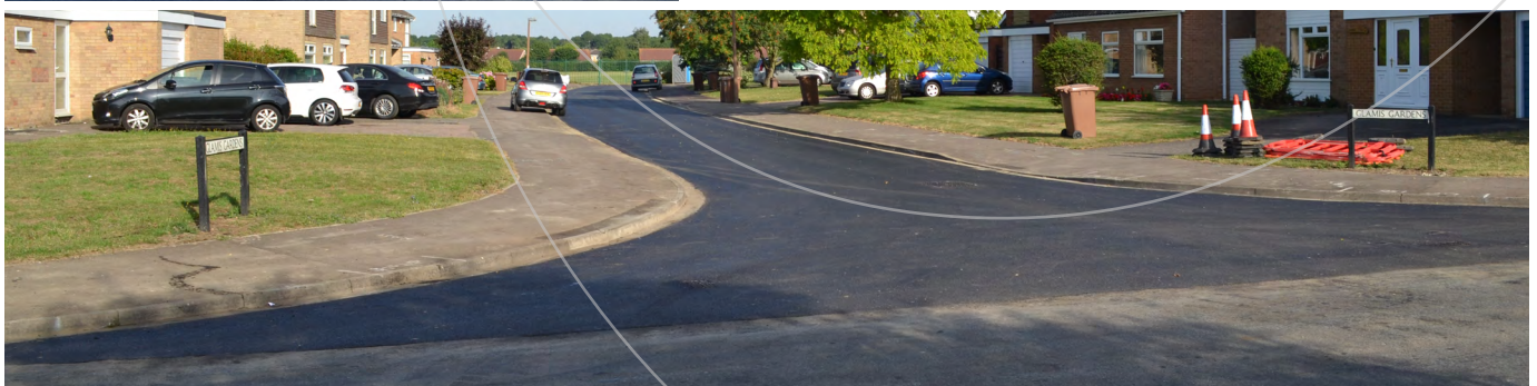
Asphalt finishing surface
