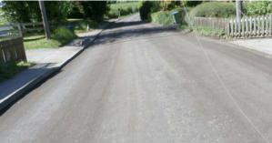
To complete the scheme Eurovia carried out the installation of a 60mm asphalt binder course which subsequently received Surface Dressing.
