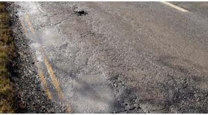
On initial visits surface issues indicated that structural failings were apparent and likely to be related to adjacent drainage and tree roots. As such, a composite geogrid system was installed on top of the recycled "SPL Stabilcourse" as an enhancement to these sections.
