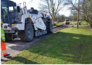
Whilst In Situ Recycling is not a new process and has been used across the UK, in line with existing Design Guides, namely TRL 386 & 611; its full extent and associated cost of the process was not regarded as appropriate for the nature of the roads under review. As such, the achievement in Cambridgeshire centres on the adaption of this process to suit the specific requirements of the local network, whilst maintaining the core benefits of this sustainable approach toward maintaining highways.
